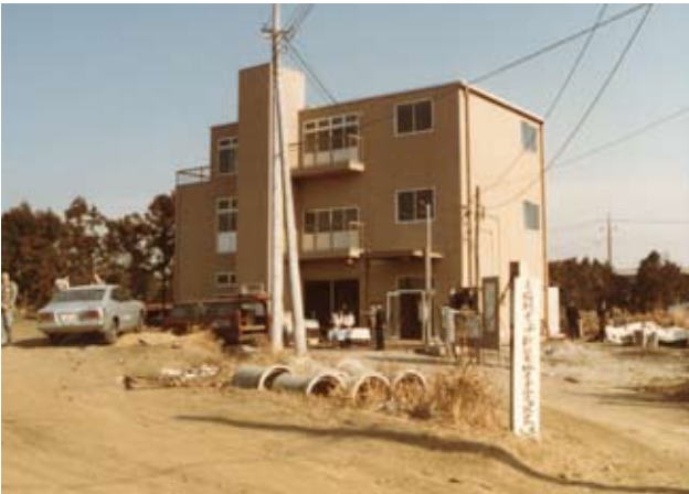
In 1984 a three-story building was completed at Yoda, Fujisawa. Later a large turning point visited us.
